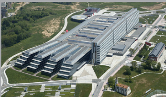
Hospital Universitario Central de Asturias Asturias, SPAIN
