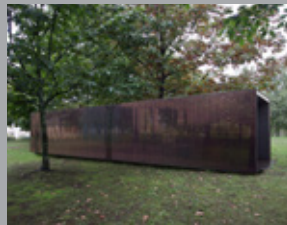
House + Lisbon, PORTUGAL
